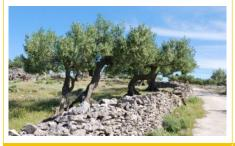
Farmland dry stone walls are man-made linear elements used as field boundaries to restrict livestock movement and/or to separate property. They are typically built using stones removed from fields and traditionally they are built of stones only, without the use of mortar. In Croatia, they are typical for the Mediterranean (coastal) region but they can also be found in some other parts of Croatia.
