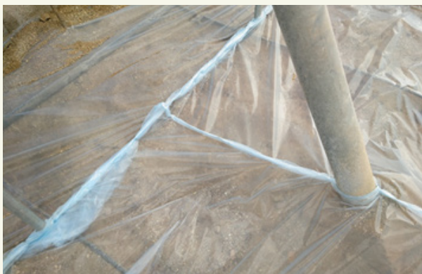
Fig. 4: Sealing of film layers can be carried on by stapling.
