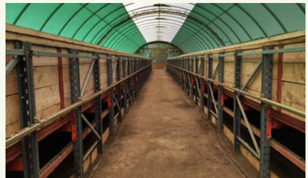
Fig. 2: Continuous flow, indoor vermicomposting facility, Austria.
