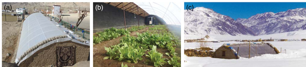
Fig. 6.8. Passive solar greenhouse technology. (a) Detail of greenhouse construction; (b) vegetables growing in the middle of winter; (c) even when covered in snow, the passive solar greenhouse functions. (From LEHO under the Geres project.)
