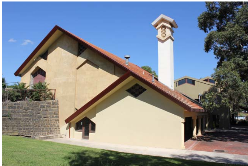
Plate 1: The Essendon Incinerator in Melbourne opened in June 1930, designed by Eric Nicholls, the first of thirteen municipal waste incinerators constructed using Griffin-Nicholls designs (the waste loading door is to the left on the upper level).
