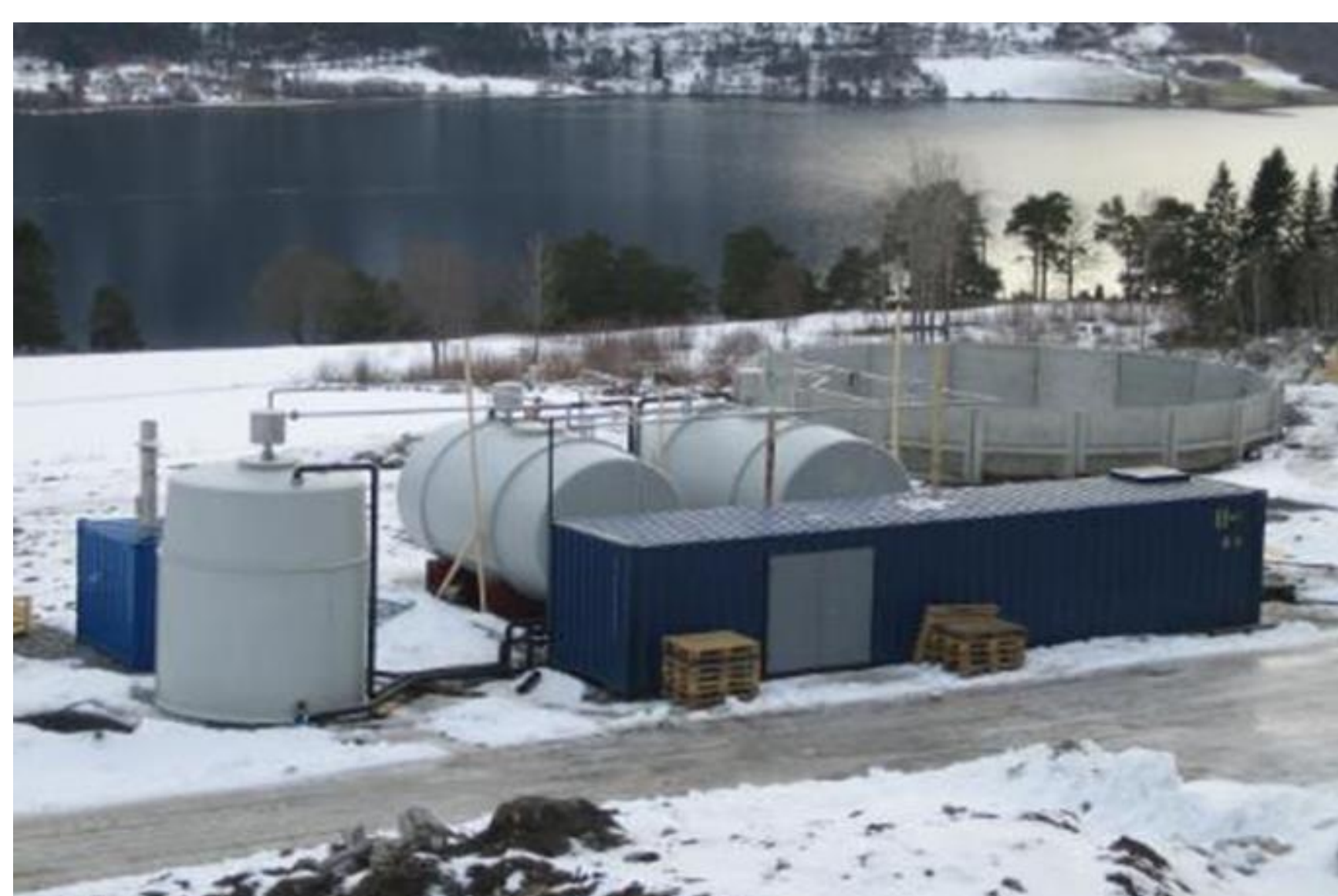
Fig.2. Biogas plant under construction in 2010, Tingvoll farm, Norway.
