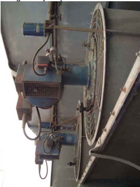
Figure 1: Looking up at the air Intake for Grain dryer
