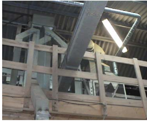
Figure 4: Elevator tubes taking grain from one piece of equipment to another
