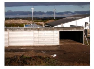
Solum 's AIKAN-plant near Holbæk. Each 600 m3 compartment is used for biogas production followed by composting of the degassed material.
