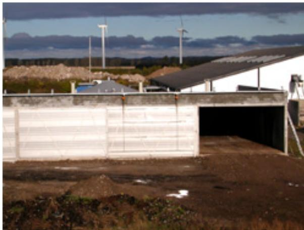
Solum's AIKAN-plant near Holbæk. Each 600 m<sup>3</sup> compartment is used for biogas production followed by composting of the degassed material.
